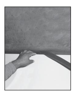
RectorSeal Blaze Foam is simple to install for head of wall applications. Compress the Blaze Foam into the joint between the top of the wall and bottom of the deck so that the intumescent strip is facing the wall surface. RectorSeal Blaze Foam can be recessed into the joint or installed flush with the outside surface of the wall. Joints are butted together. No mechanical fastening of Blaze Foam is required.
