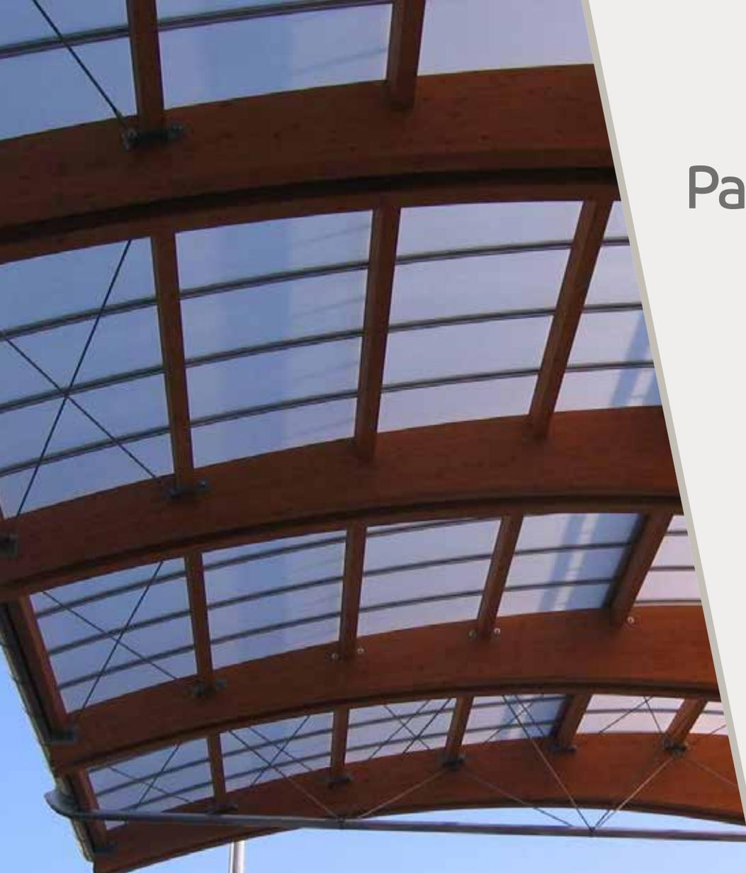
A photograph of a curved aluminum truss structure supporting a translucent polycarbonate roof. The structure is made of brown-painted metal beams and cross-bracing, set against a clear blue sky.
